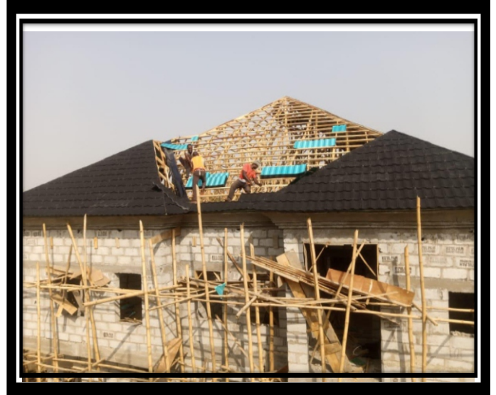
Work in progress in Life Camp, Abuja
