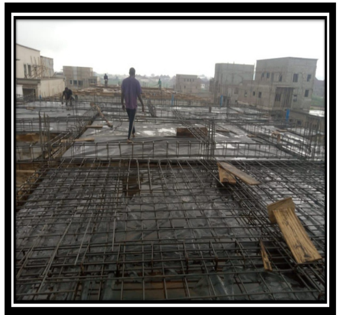
Workers on site at Lokogoma, Abuja
