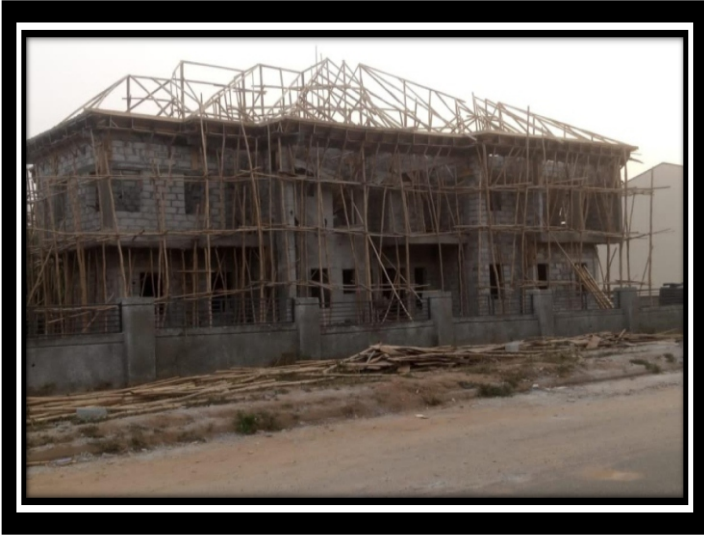
Construct site at Ensica Real Homes Estate, Abuja
