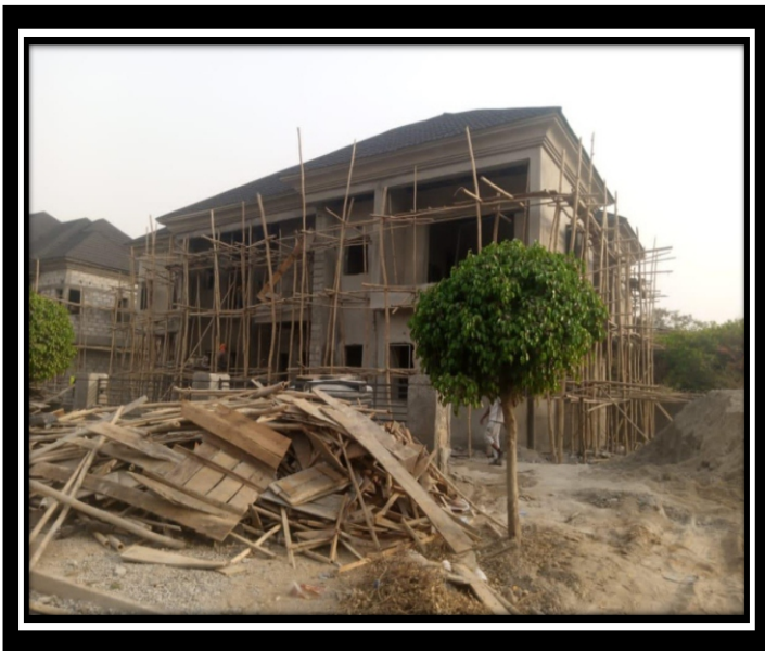
Our site at Apo, Abuja (work in progress)
