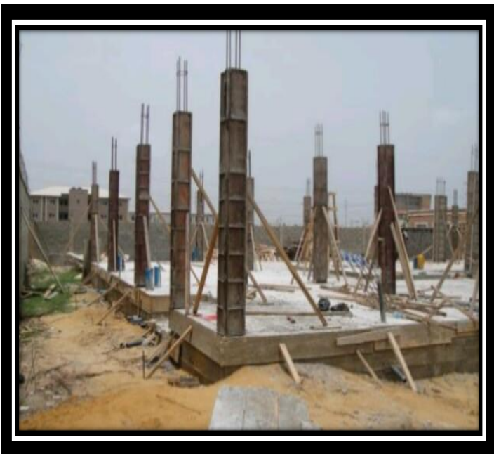
Work in progress on a foundation at Apo
